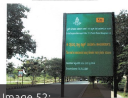
Image 52: Asphaltting of roads
